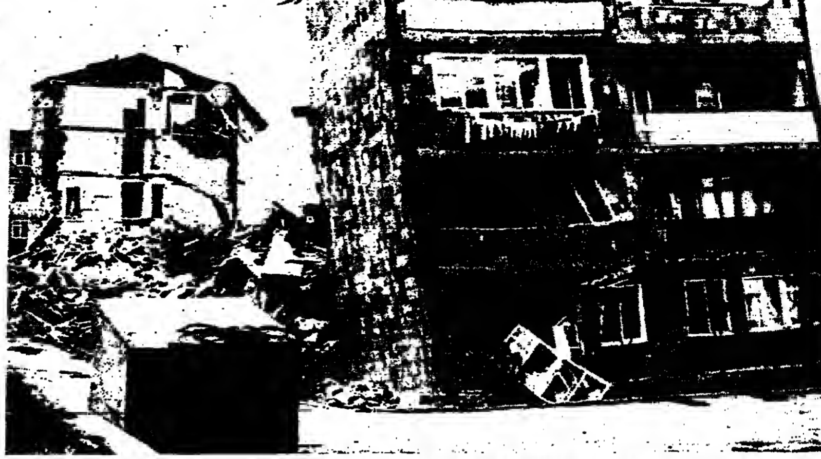
Apartment blocks reduced to rubble or left leaning dangerously off-centre in the town of Spitak, one of the areas in northern Armenia worst hit by the quake.
